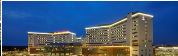
Adana Integrated Health Campus, Turkey: integrated security system to protect the entire campus
