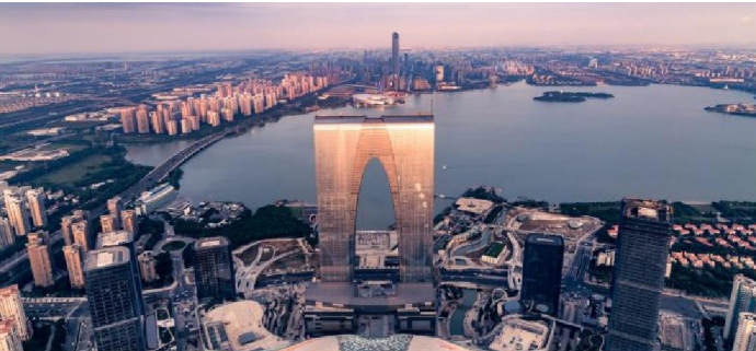
Suzhou Center: Future-oriented security for cutting-edge multi-purpose complex in China
